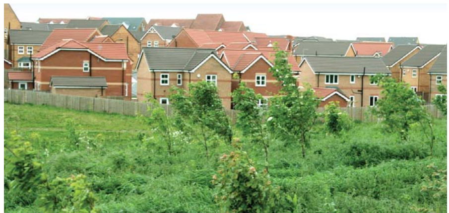
The houses at Silverwood no longer look onto a desolate grey scar
